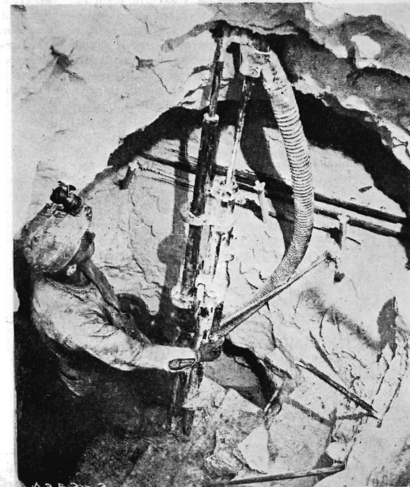
The same miner drilling with dust control equipment. This picture was taken with the same camera and the same camera setting as the one on the opposite page. (Both photographs courtesy of Kadco Corp.)
