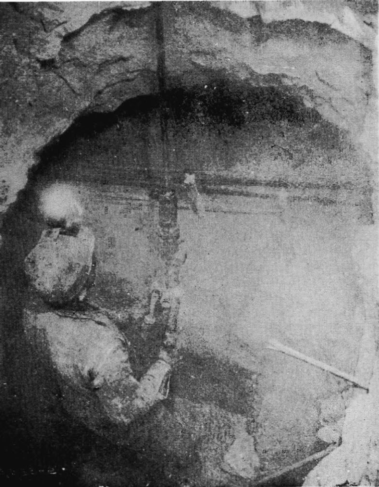
A mine worker drilling through rock without dust control equipment. The air is thick with the silica-laden dust that causes the fatal anthraco-silicosis.
