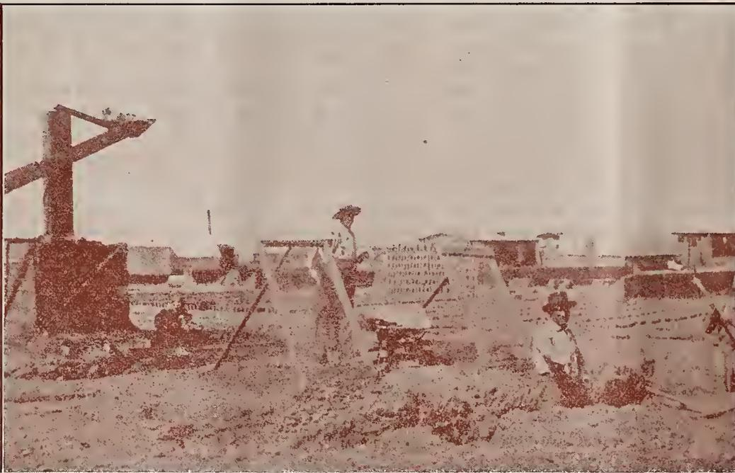
Making Clay Bricks. Note "Pug Mill" and Some Completed Houses
