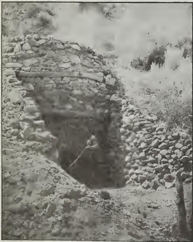
Burning Limestone for Material Used in Concrete Construction at Llano del Rio
