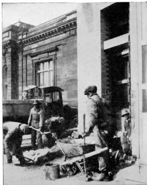
1. Negro laborers doing construction work on Taylor Hotel, Akron, Ohio.
