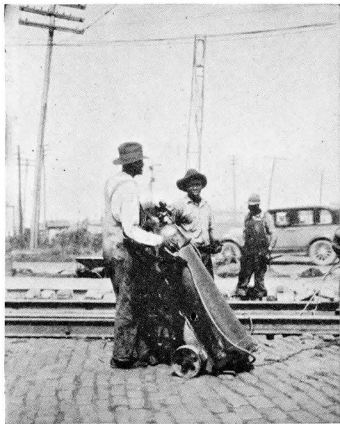
13. Negro welders working on street railway, Norfolk, Va.
