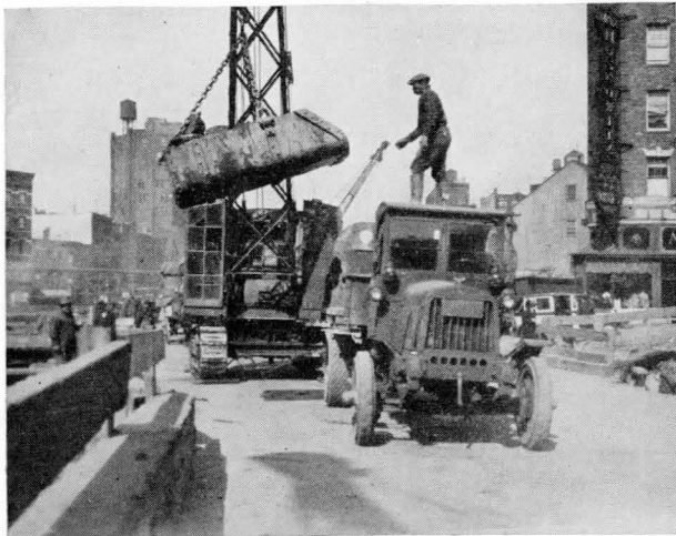
16. Negro worker handling rock from New York subway excavation.
