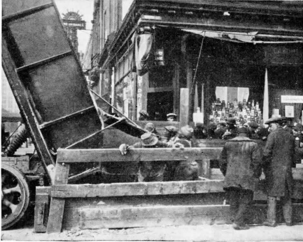
15. Negro workers on Philadelphia subway, pouring cement.
