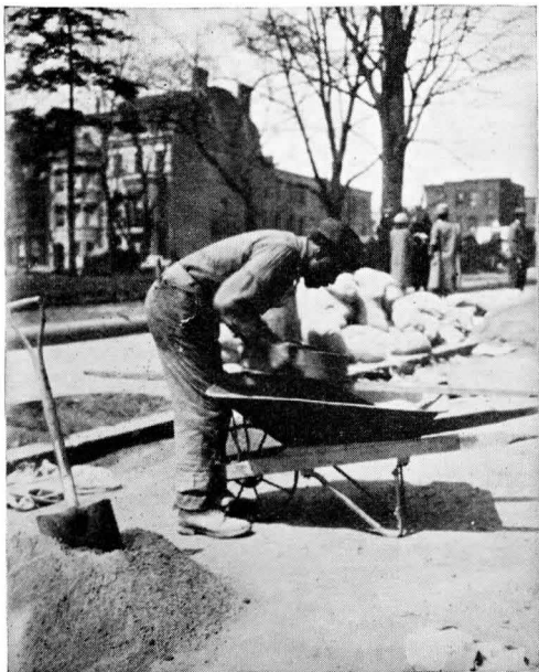
11. Negro worker on street construction job, Washington, D. C.
