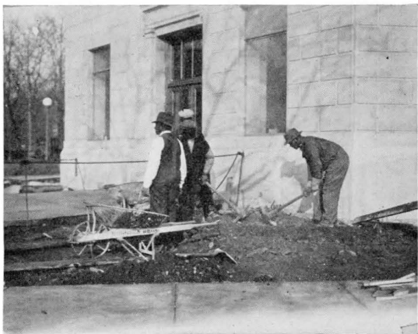
9. Street paving work, Washington, D. C.
