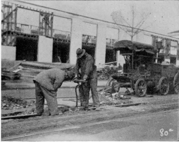
7. Negro workers in Washington, D. C., relaying the street railway.
