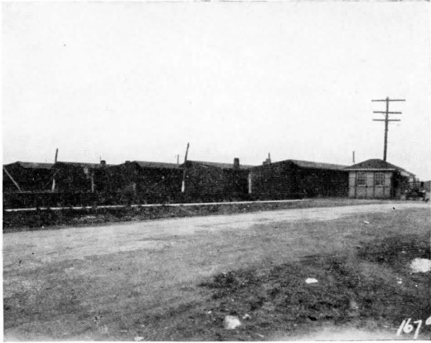
23. Barracks provided by Bethlehem Steel Company for Negro workers, Sparrows Point, Md.
