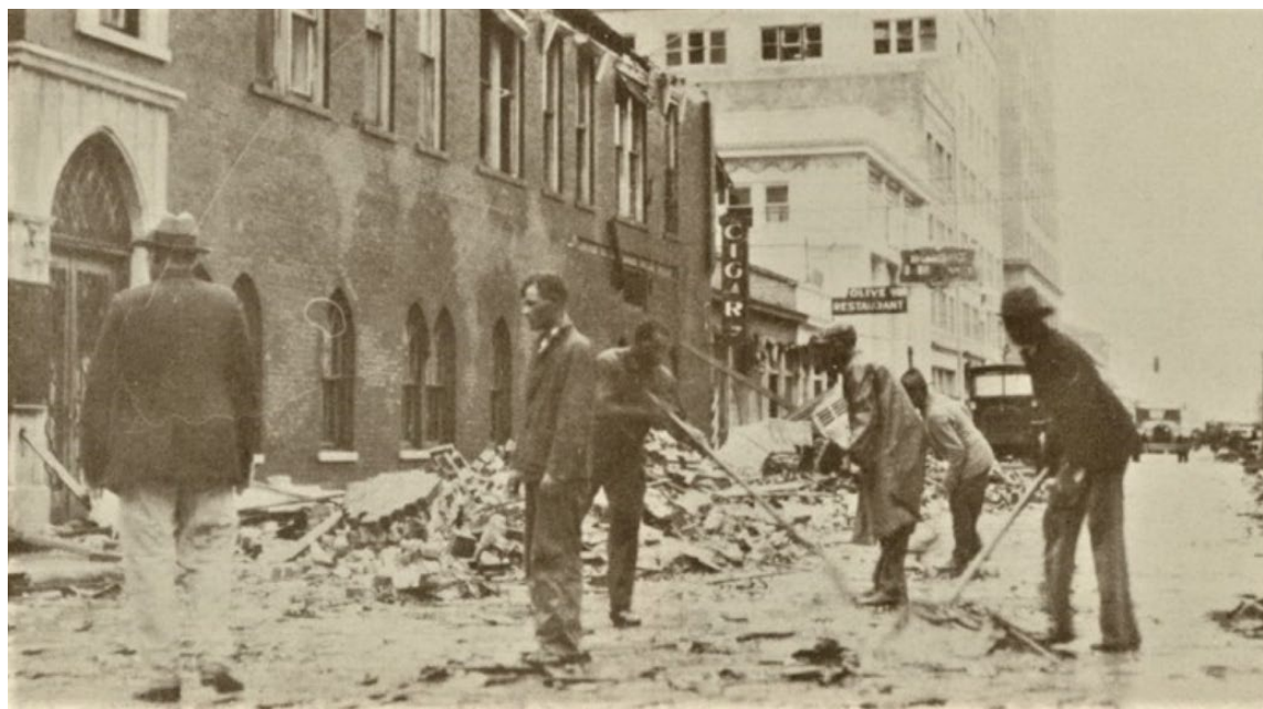
Clearing Olive St. in West Palm Beach.
