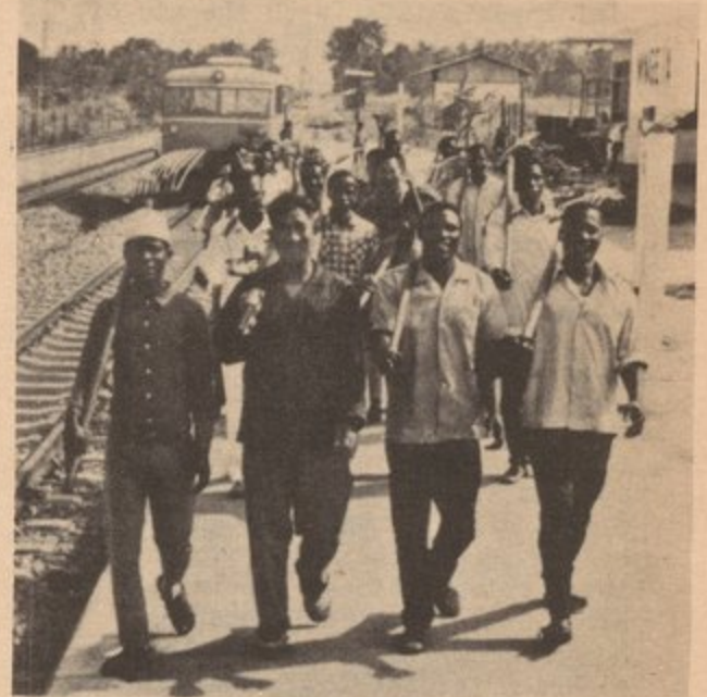
Tanzanian, Chinese and Zambian workers set out to build the Tanzam Uhuru Railway. (Photo: Tanzanian Embassy)
