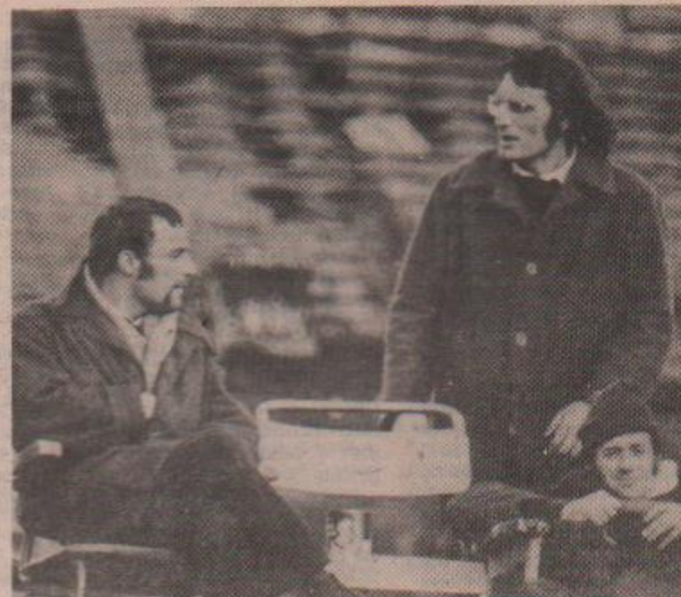
Some of the prisoners with damaged roof (behind)
