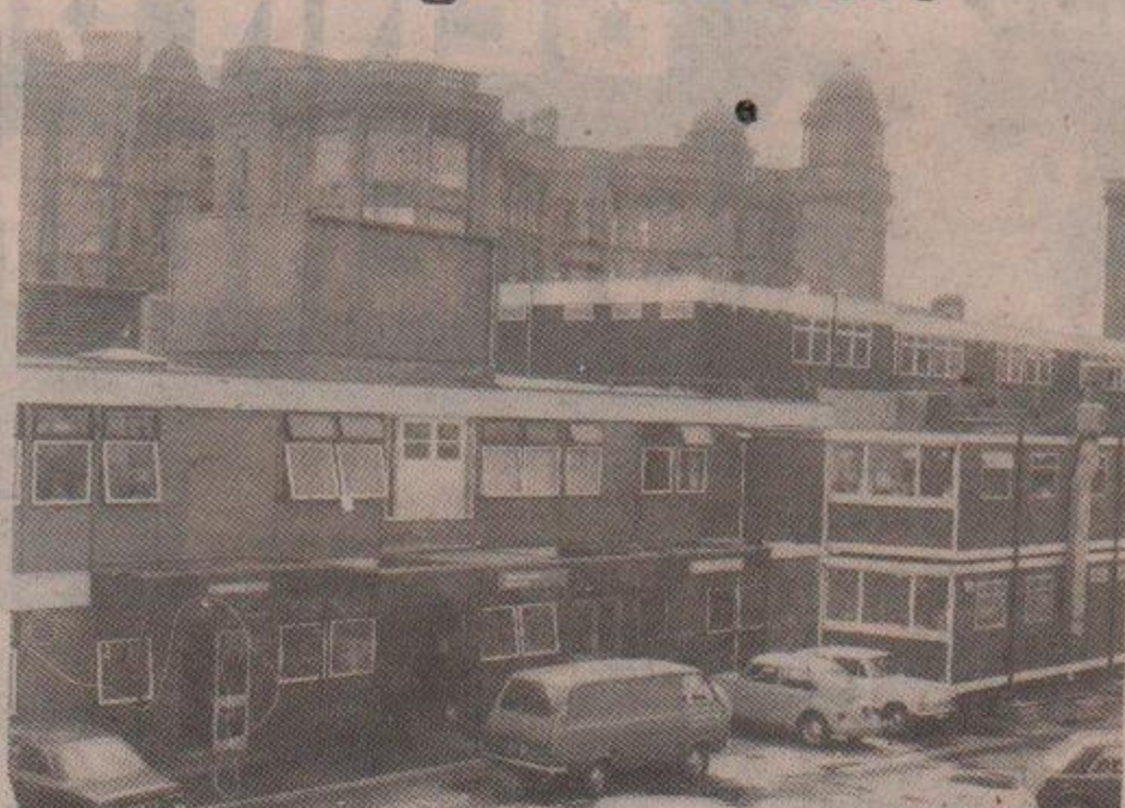
Portable cabins are now used to supplement the inadequate Glasgow hospital buildings
