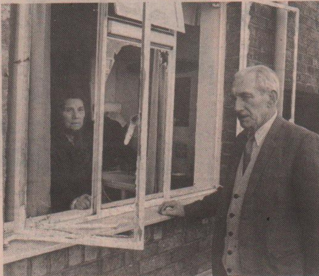
William Stills, who lived only three houses along from the explosion was fortunate to escape injury. He was reading at the kitchen table. The blast shattered the windows with such force that the glass flew over his head and into the wall opposite. The door was wrenched off its hinges and blown into the house. Mr Stills, pictured above with his wife, said that if he had been standing up he would have been badly cut, at the least.
