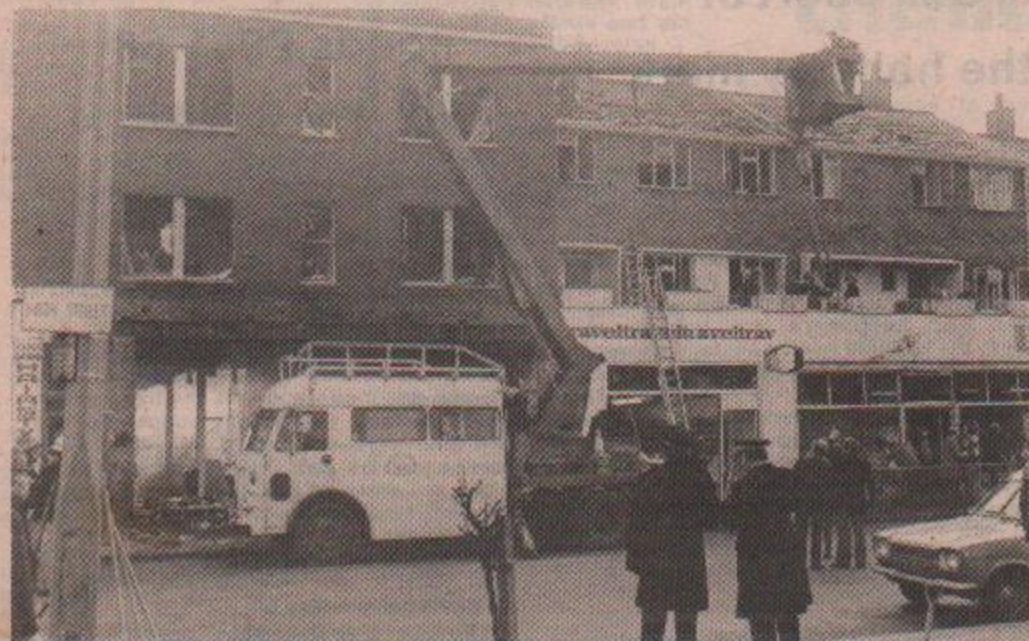
Widespread damage — in Brentford High Street following the blast in Stones' men's-wear shop
