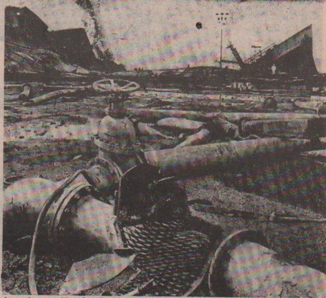
Large pipes were blown from the ship with such force they became embedded in asphalt.
