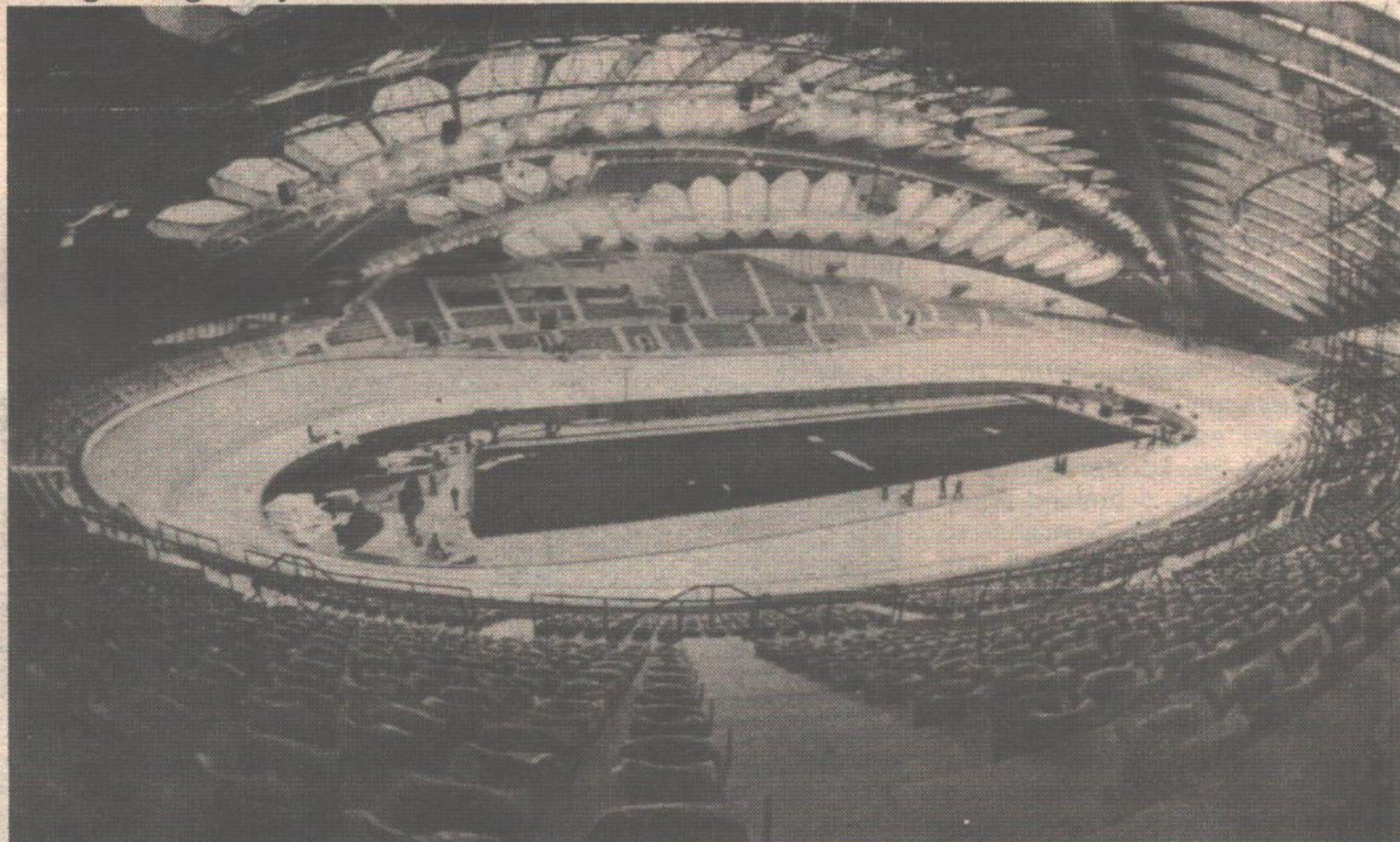
The Olympic Velodrome leaks when it rains
