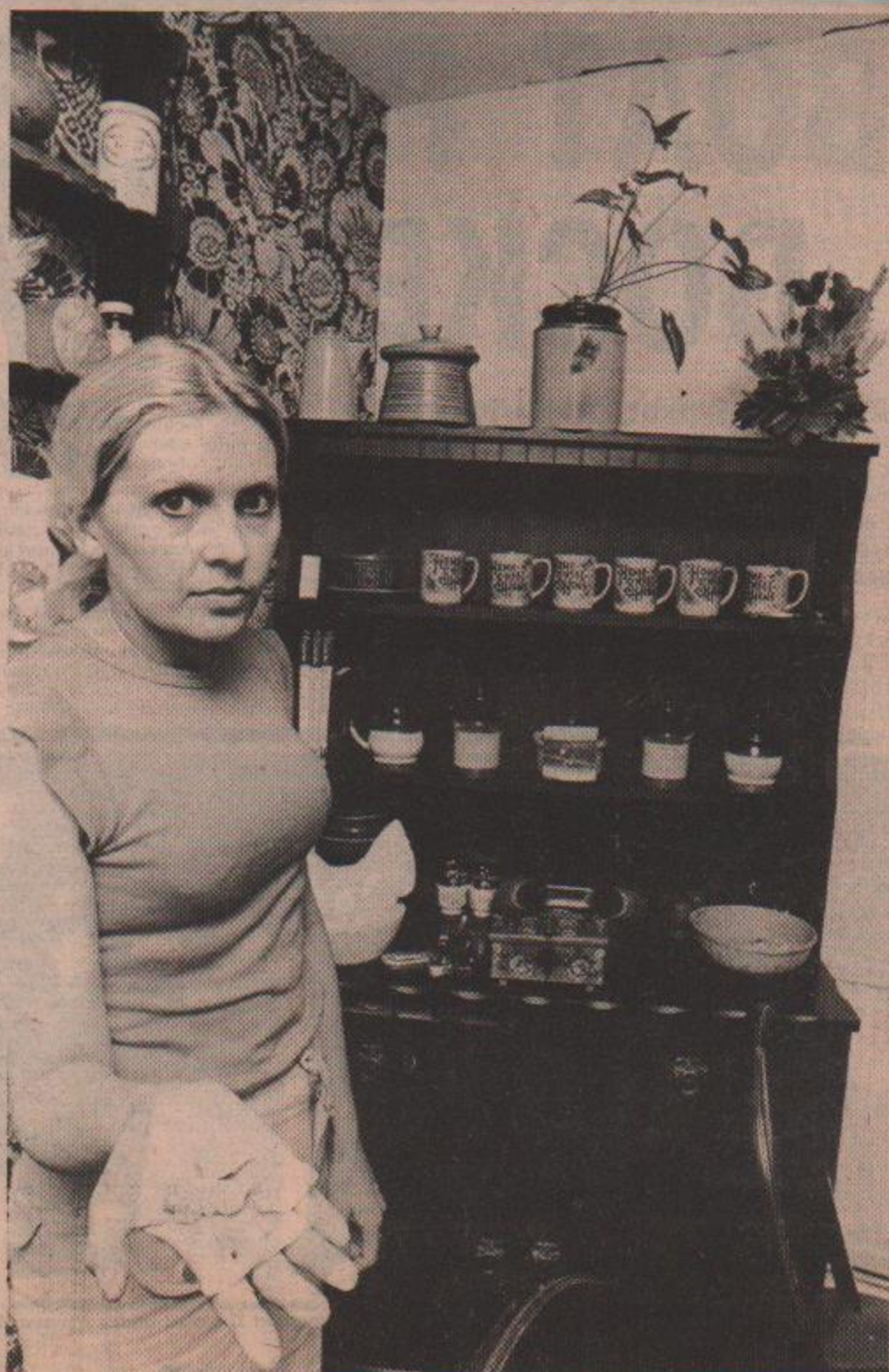
MRS SANDRA ASHBY holds pieces of plaster that have fallen from the joints between wall and ceiling in her dining room
