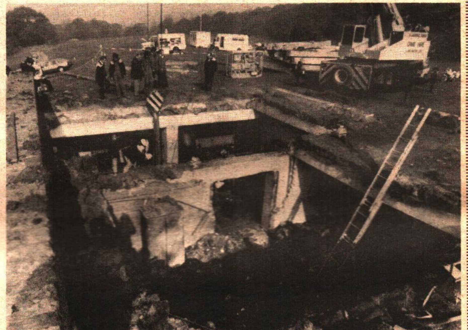
100 tonnes of concrete of concrete girders and earth were lifted into the air
