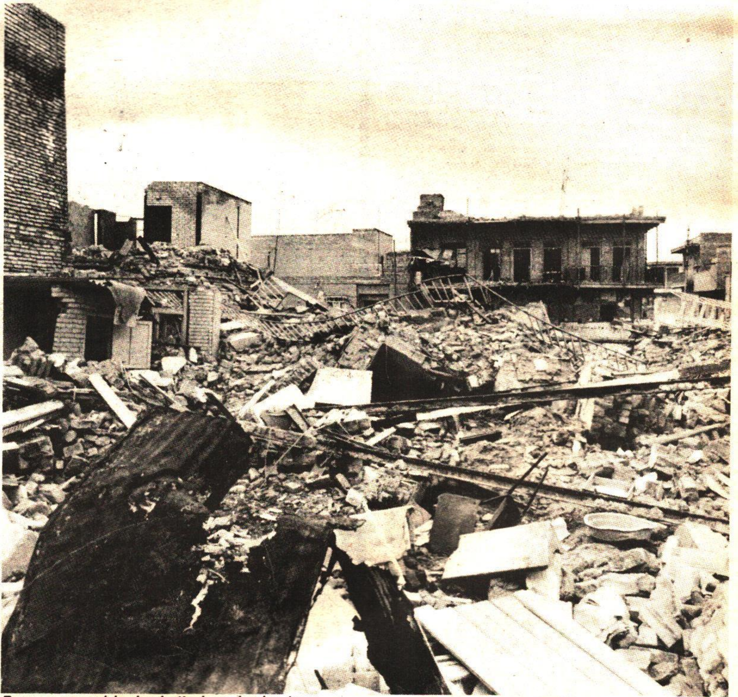
Damage caused by Iraqi attack on Iranian town
