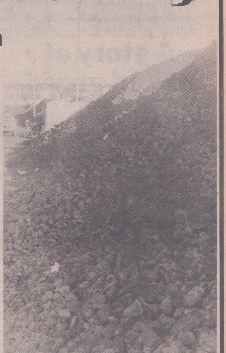
THE COAL stocks are so high either side of the road running through Ravenscraig plant that it has become known as the 'Grand Canyon'
