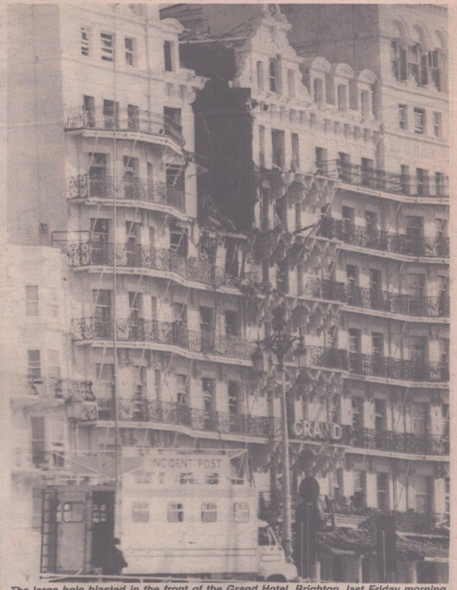
The large hole blasted in the front of the Grand Hotel, Brighton, last Friday morning
