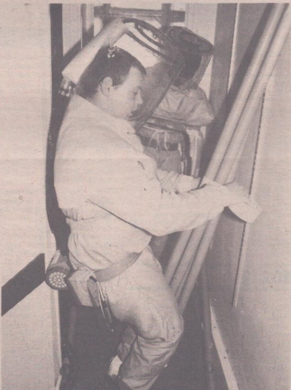
Lambeth council workers using special equipment for the safe removal of asbestos
