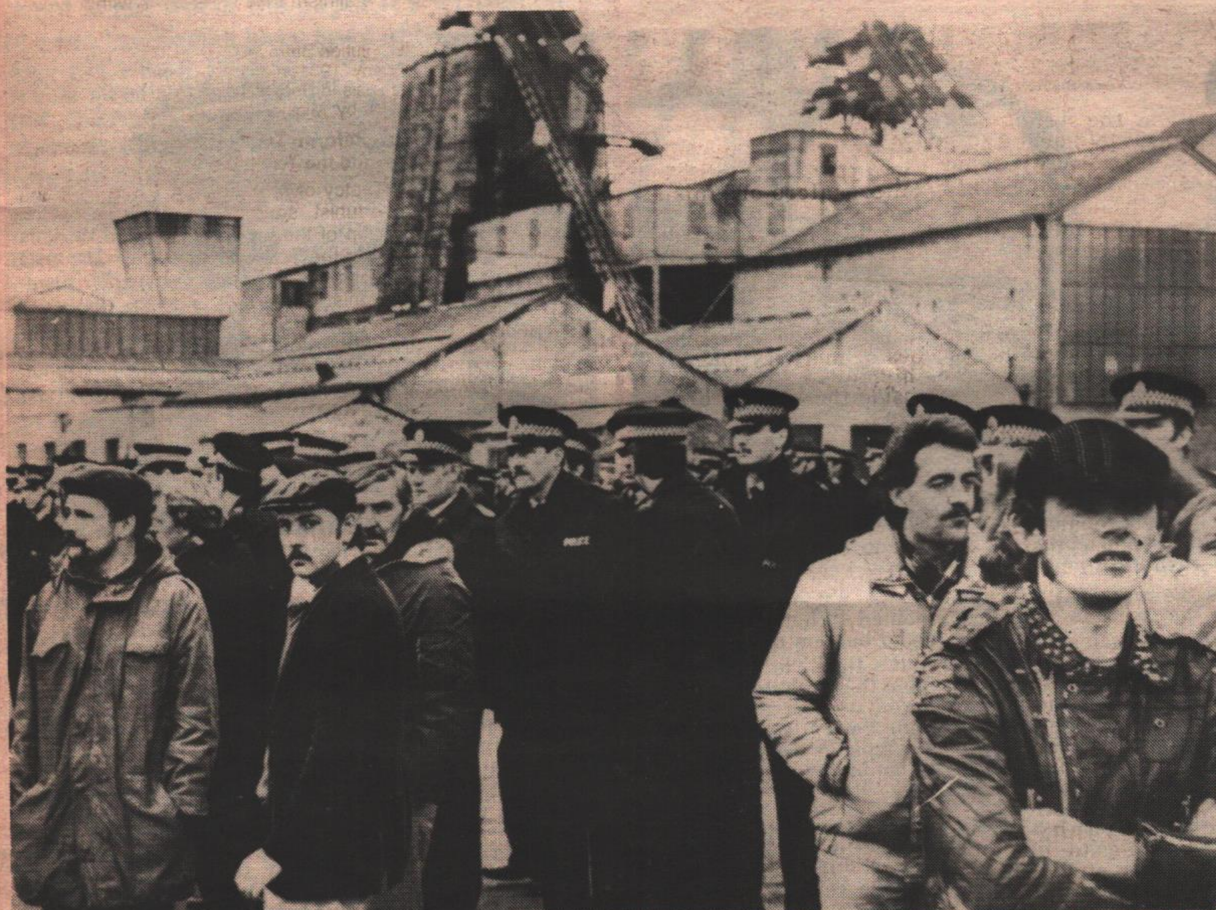
A large force of police formed up at Polkemmet pit yesterday, separating pickets from scabs
