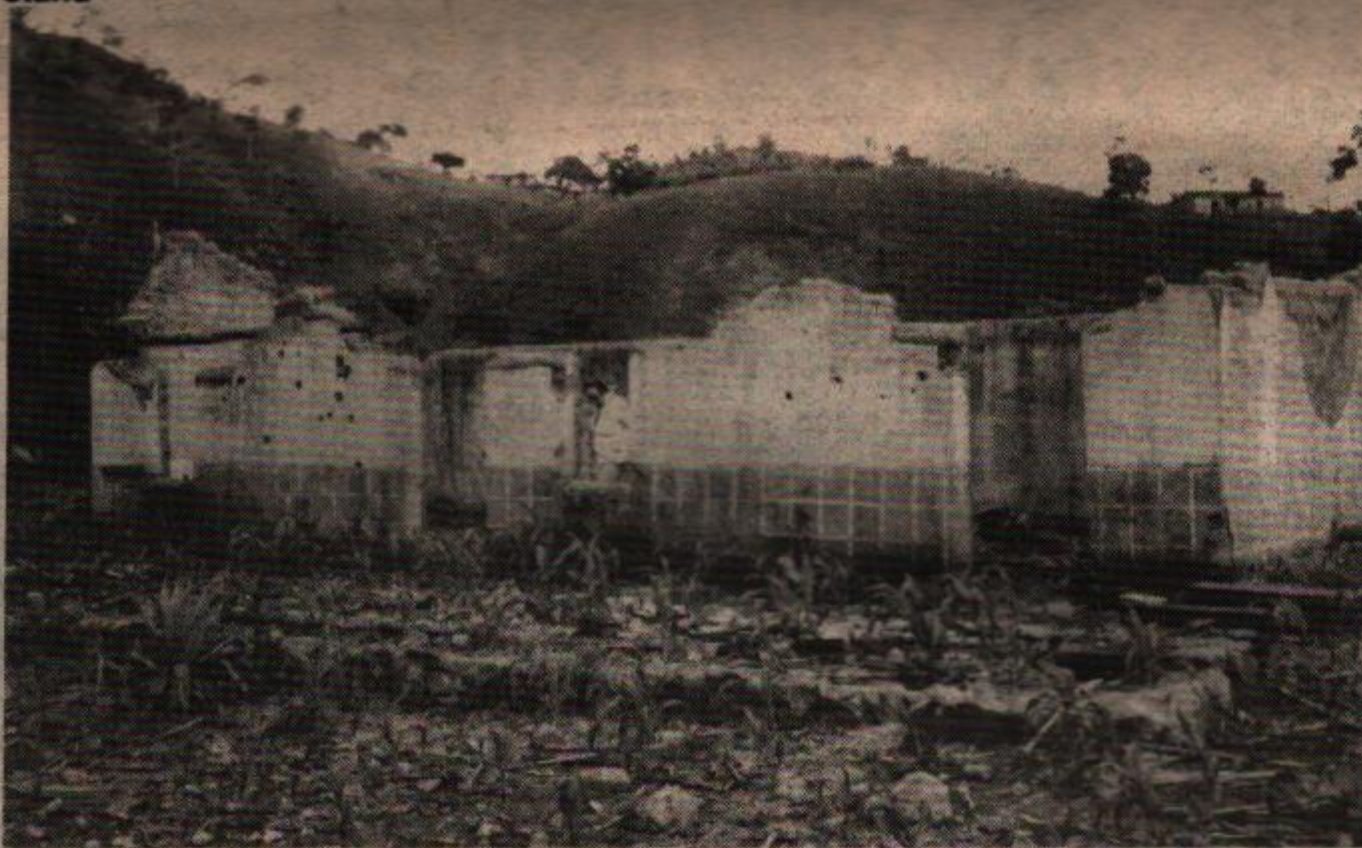
The ruins of one of many bombed-out school buildings outside San Salvador
