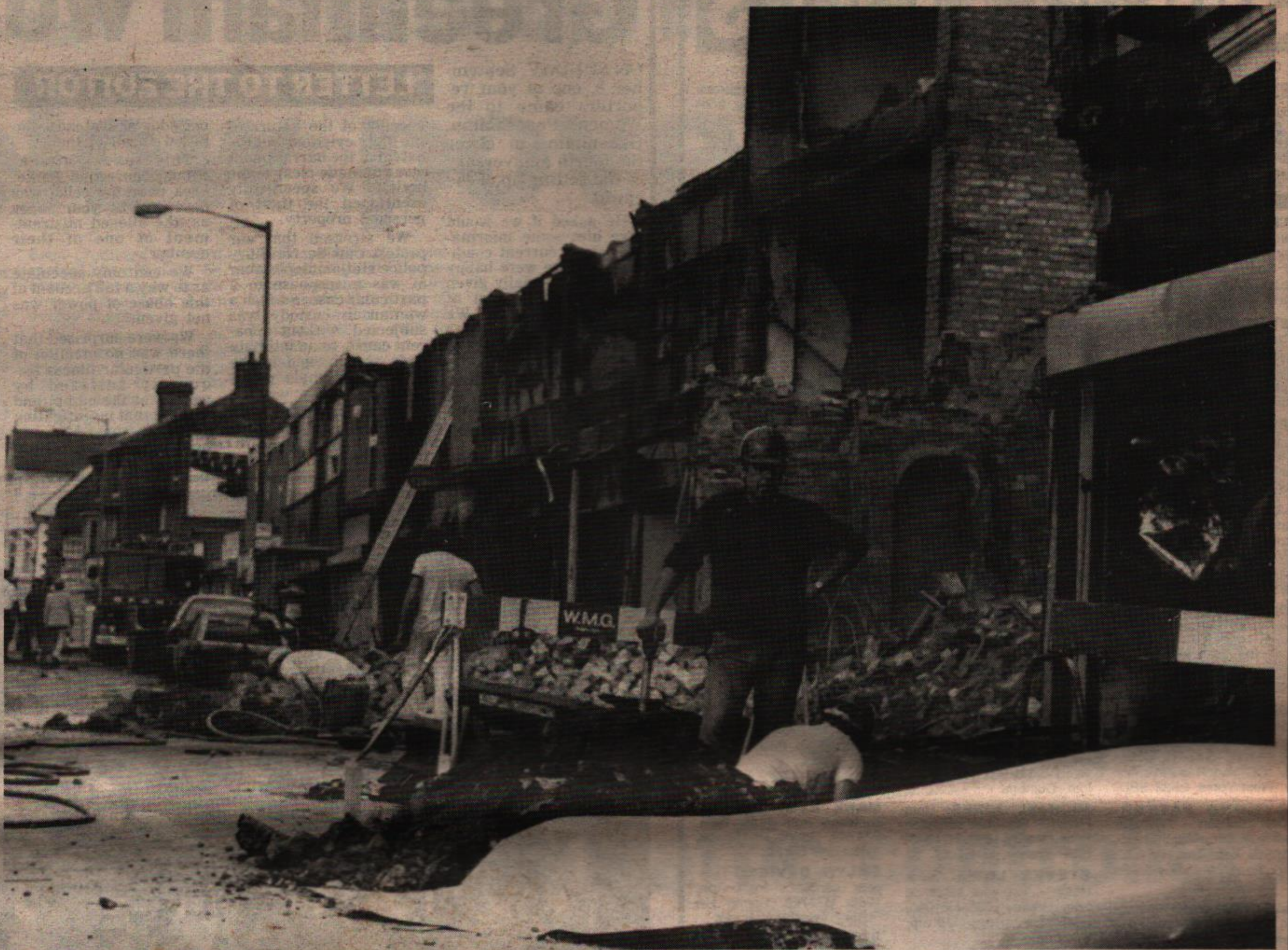
Clearing up operations underway in Lozells Road
