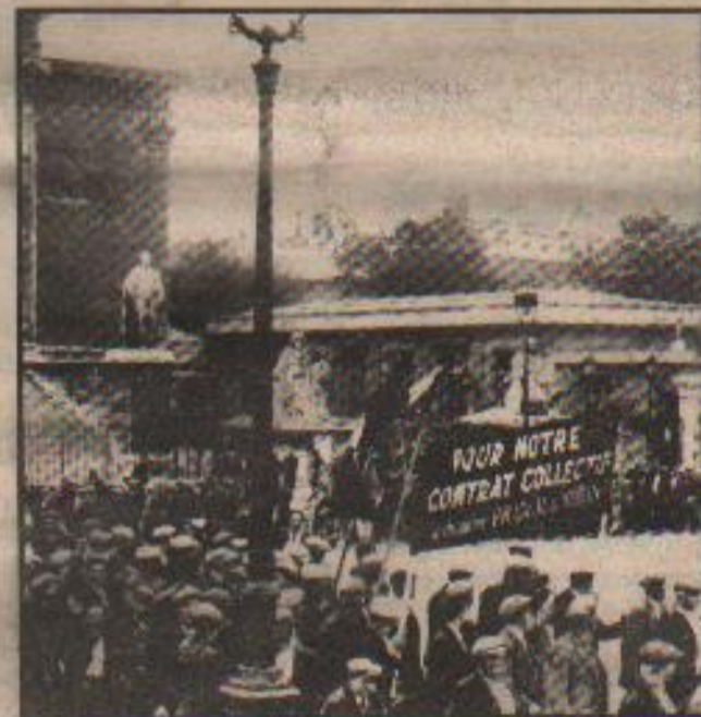
1936: building workers march on the parliament building after the election of the Popular Front Government.
