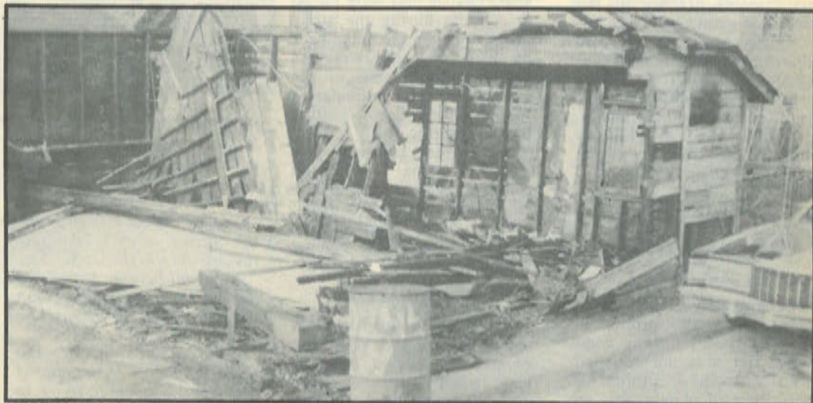
Dudley Emmons garage was burned to the ground
