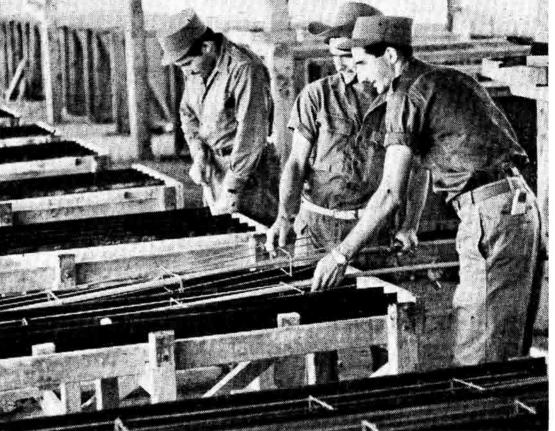
In the photo above, three soldiers place rods in forms for concrete slabs. When finished these will be put together to make walls and roof.
