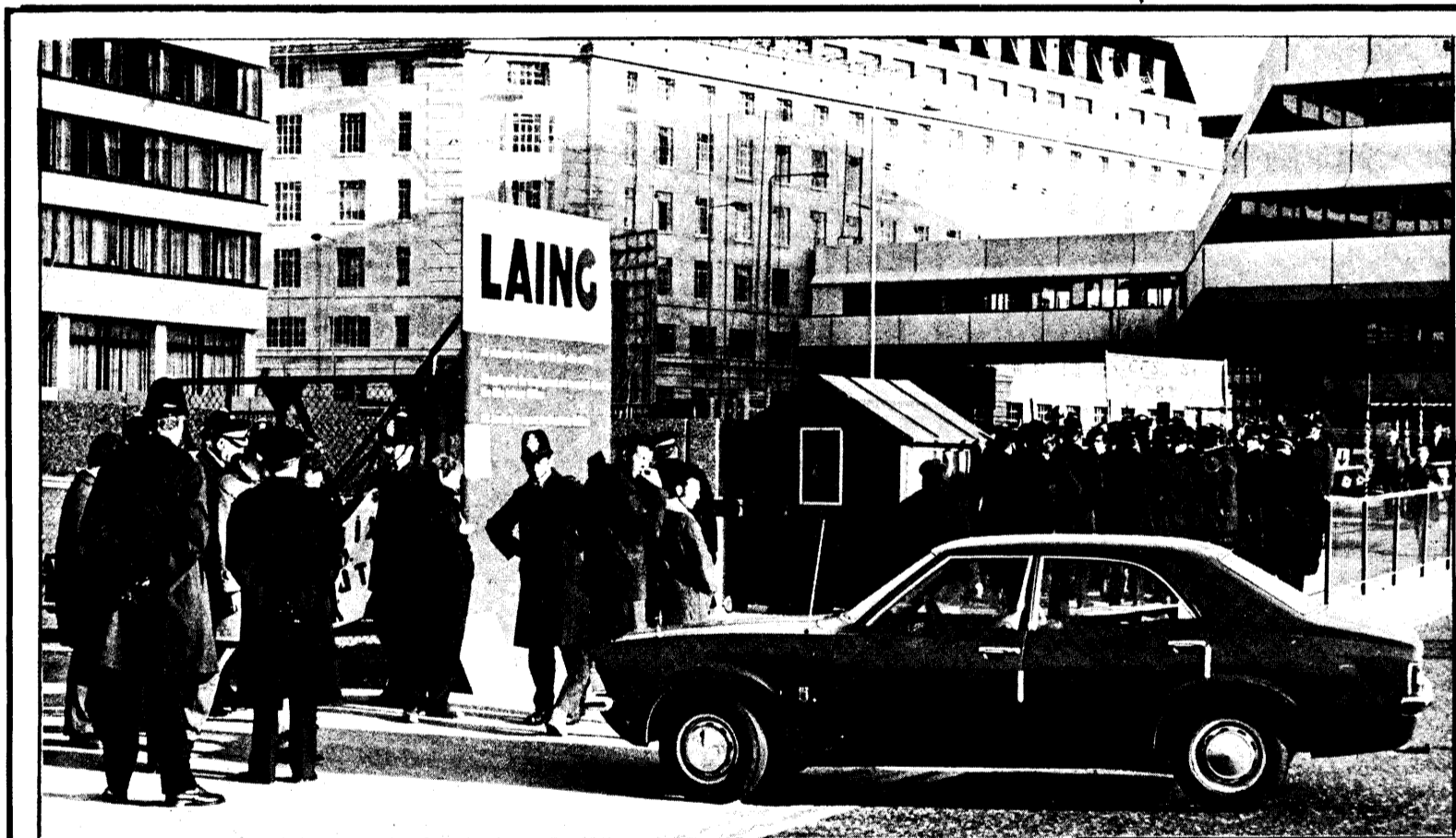
AN ANTI-PICKET squad again swamped builders and electricians protesting outside the St Thomas' hospital site yesterday ● See story page 3.
