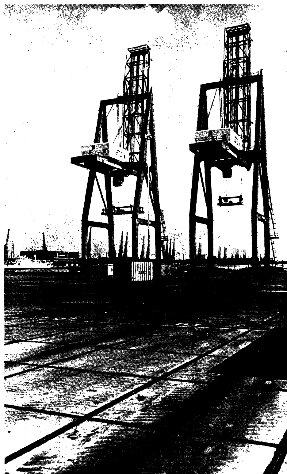
With the development of monster gantry cranes (left) and straddle carriers, cargoes previously shifted by 100 men in two weeks are now moved in containers by 13 men in 24 hours—or less.
