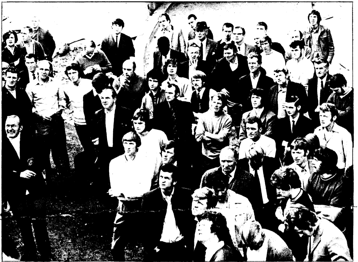
Preston building workers out on mass picket
