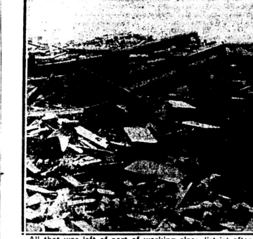
All that was left of part of working class district after storm hit West Frankfort, southern Illinois coal mining town.
