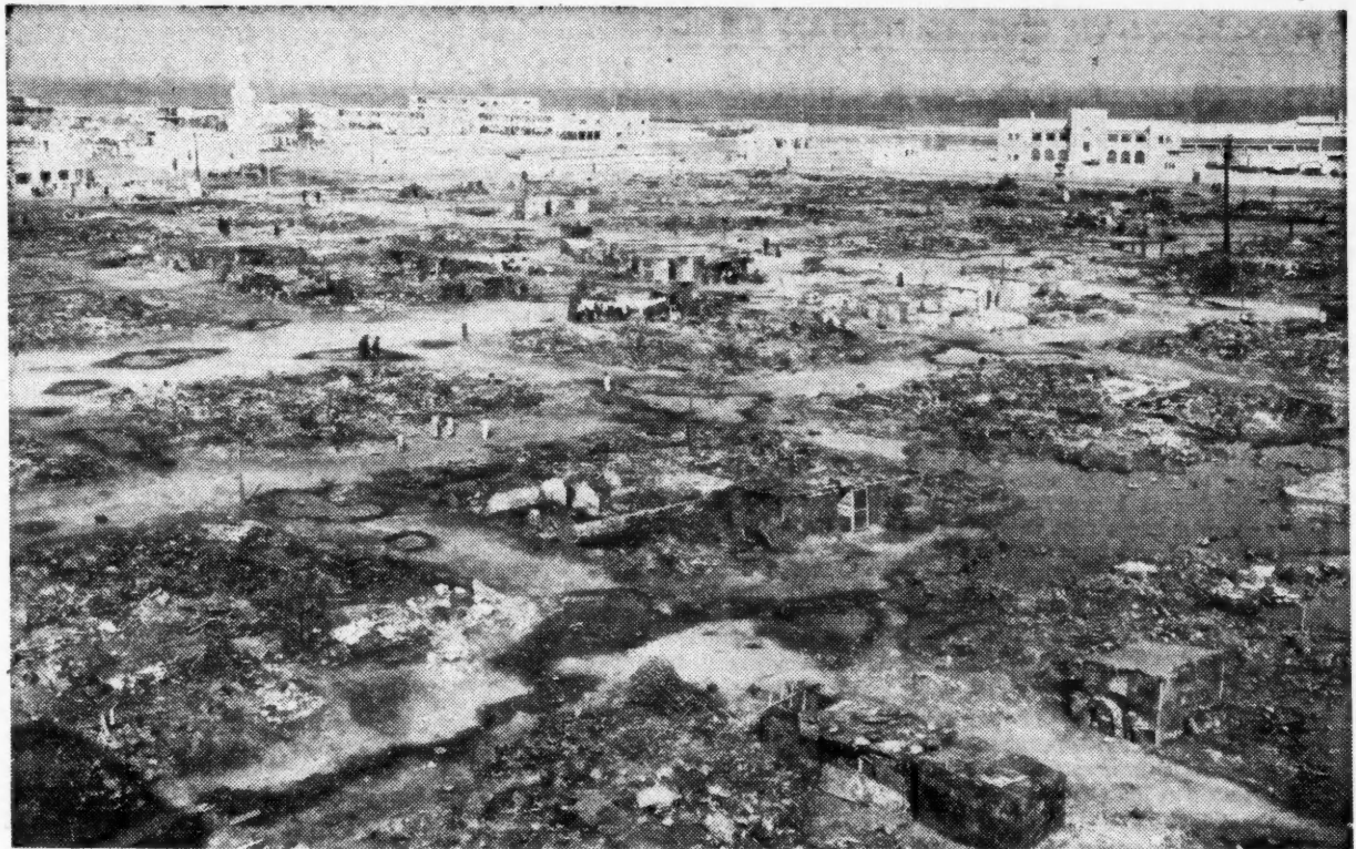
THIS WAS THE "NATIVE QUARTER" OF PORT SAID AFTER THE ANGLO-FRENCH BOMBING It covered 40 city blocks of homes and shops—and it makes understandable Egyptian hatred of imperialism
