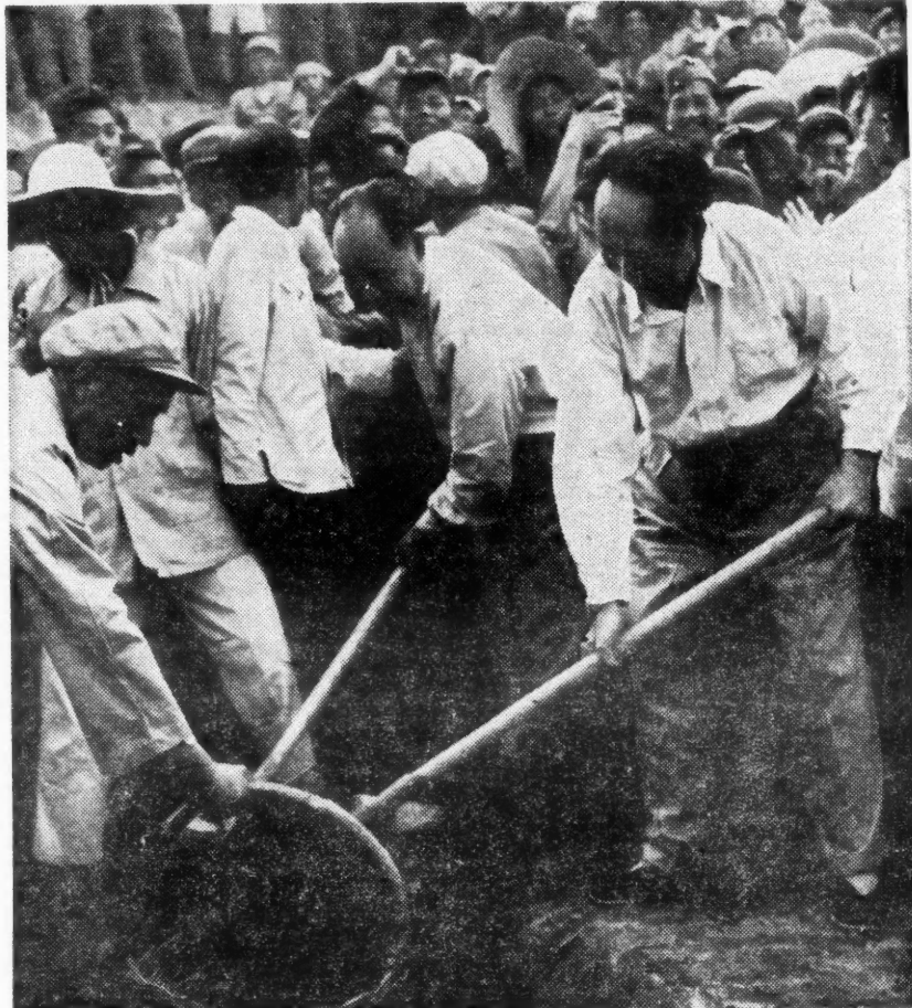
EVERYBODY WORKED TO BUILD THE MING TOMBS RESERVOIR Chairman Mao Tse-tung himself (right) put in a full 8-hour day.
