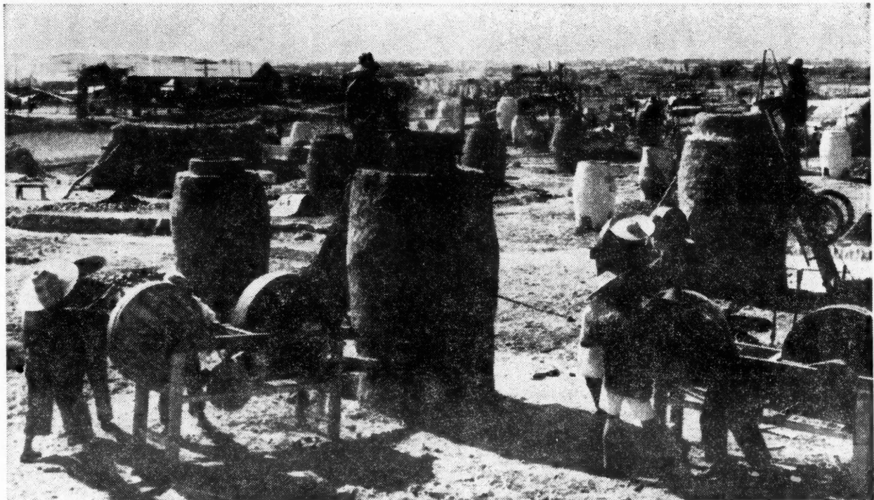
STEEL FURNACES LIKE THESE CAN BE—AND ARE—BUILT OVERNIGHT Many are operated with hand bellows, but some have power-driven blowers.
