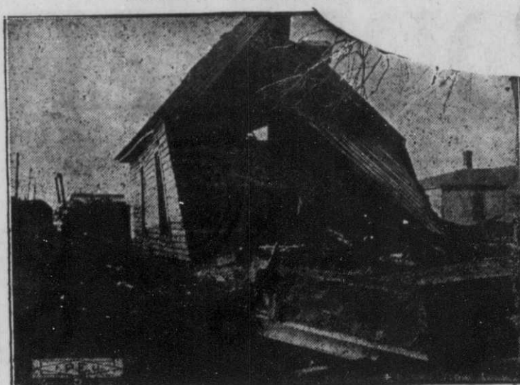
This shows the home of Joe Carso, an Illinois miner, after it had been bombed by coal company gunmen, following a gun fight between mine guards and striking miners
