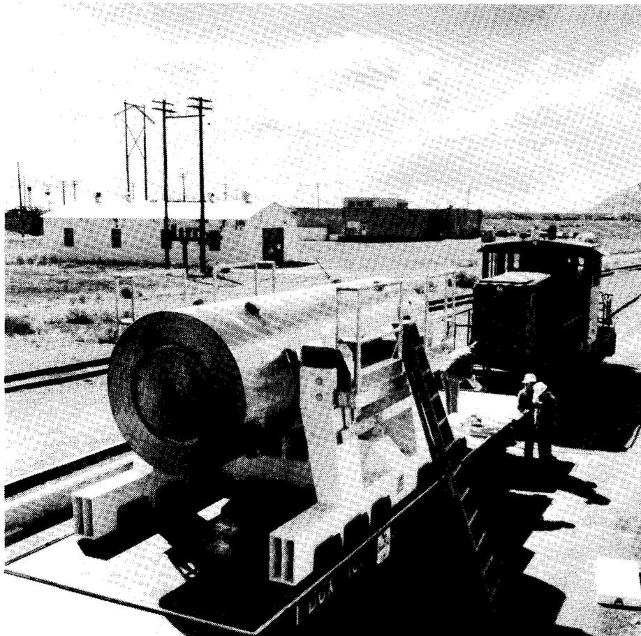
America's nuclear industry in transit: Fuel and structural core materials from TMI are shipped by rail to the DOE's Idaho National Engineering Laboratory. Photo courtesy DOE.
