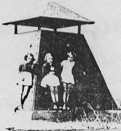
*This strange looking steel structure standing near the gate of the Bemis Textile Mill in Talladega, Ala., is being held in readiness by the mill-owners to murder their workers should they exercise their right to organize. Thugs can sit in safety inside its steel walls and poke their machine guns through the triangular openings in its sides.*
