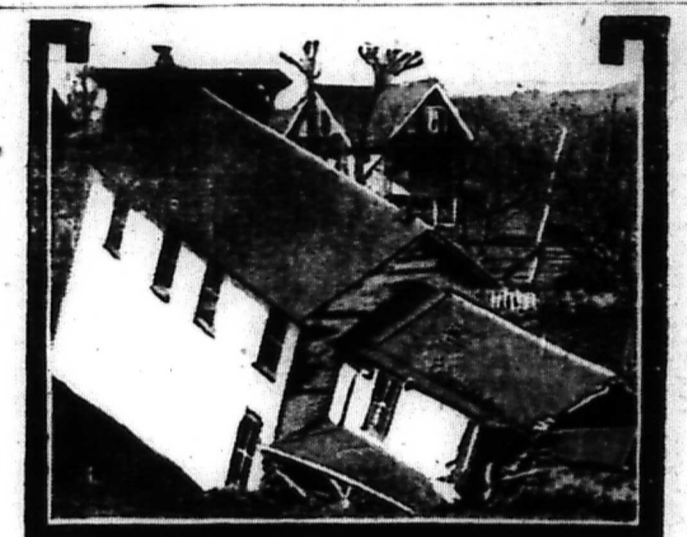
TYPICAL SCENE IN PITSTON. A HOME SINKING INTO THE EARTH.
