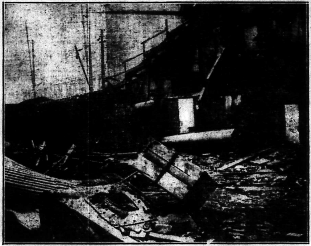
Scene of Boiler Explosion at Cordage Trust Mill.
