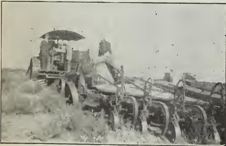
This giant tractor, with two men in charge, clears ten acres of land a day. It mows down monster "joshua" trees, greasewood and sage in an astonishing manner. These tractors are also used for digging irrigation ditches on the Llano property. It digs a ditch three feet deep and two feet wide as it sweeps steadily and irresistibly along the lines marked out by the surveyors. All of the plowing will be done by these machines.
