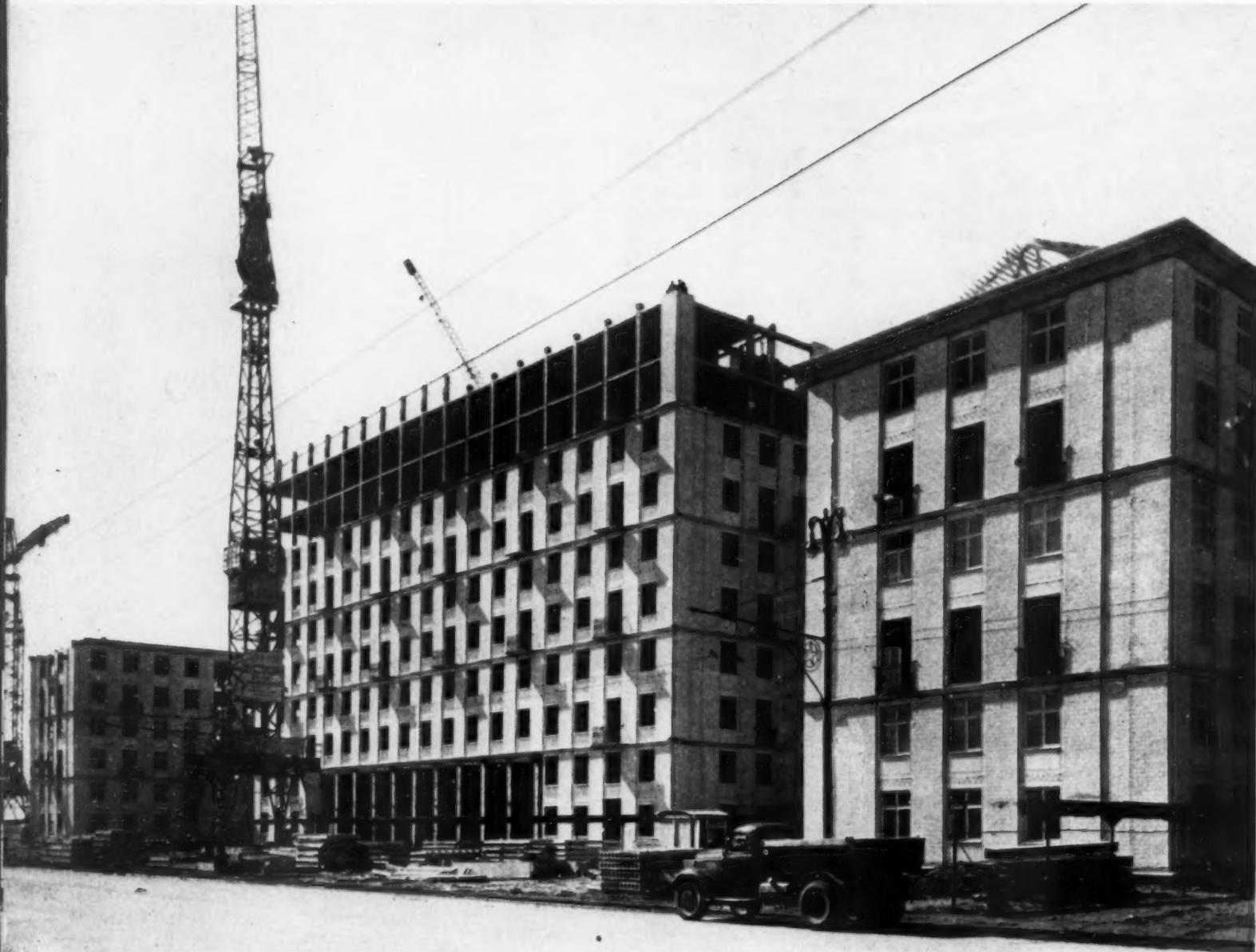
BUILDING SITES ARE BECOMING ASSEMBLY LINES. WHOLE WALLS ARE CONSTRUCTED INDUSTRIALLY AND ONLY NEED ON-THE-SPOT FINISHING. FRAMES, DOORS AND SASHES ARE DELIVERED ALREADY PAINTED AND WITH GLASS IN PLACE. OTHER SECTIONS HAVE A FINISHED CEILING FOR ONE STORY AND A FLOOR FOR THE ONE ABOVE.
