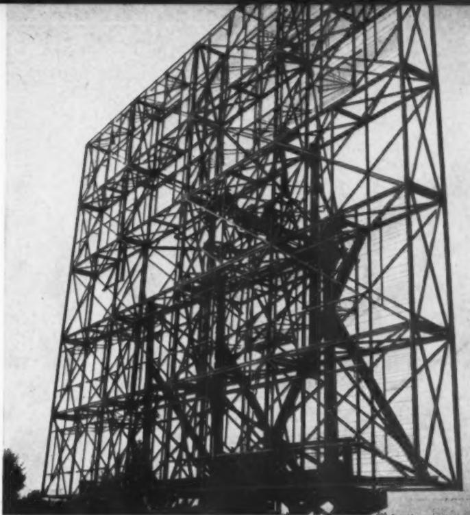
THIS STEEL LATTICE WORK IS THE ANTENNA OF A POWERFUL RADIO TELESCOPE.
