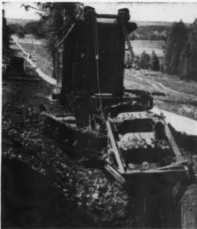
Rotary excavator cuts trench, partly through mountains, in which pipeline is to lay. The pipe sections are then welded by mobile automatic machines.
