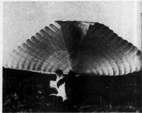
PARACHUTE RETURNS A ROCKET'S INSTRUMENT SECTION.
