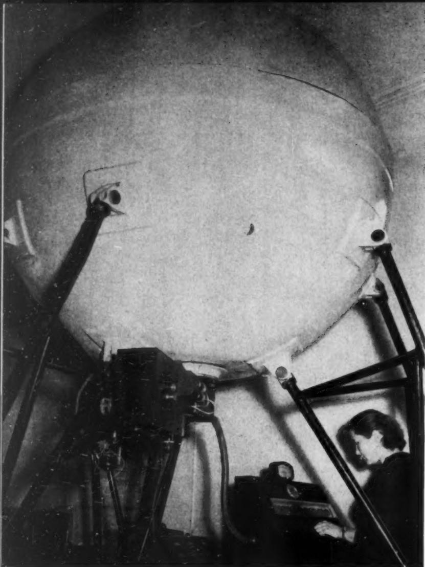
THIS IONIZATION CHAMBER RECORDS COSMIC PARTICLES PASSING THROUGH IT.
