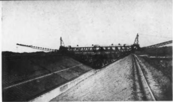
SPECIAL MACHINE THAT SHAPES AND CLEARS CHANNELS EQUALS WORK OF 500 MEN.
