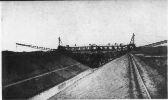
SPECIAL MACHINE THAT SHAPES AND CLEARS CHANNELS EQUALS WORK OF 500 MEN.
