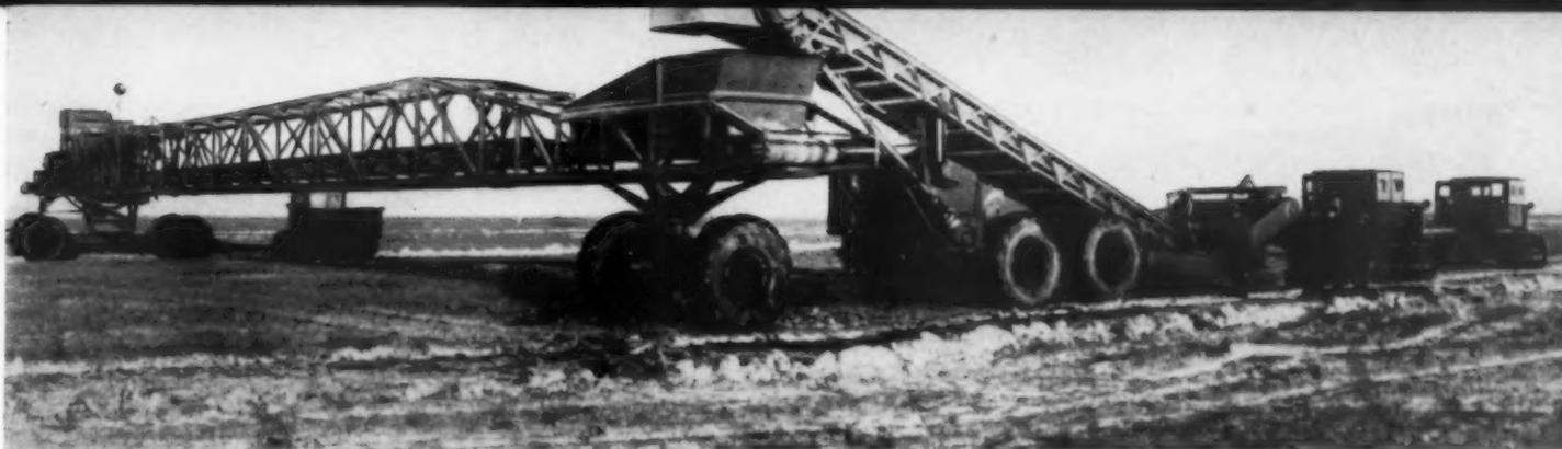
THIS GIANT EARTH MOVER FOR CANAL WORK HAS A PLOW 10 FEET WIDE, A CAPACITY OF 1,960 CUBIC YARDS PER HOUR AND DUMPS ITS LOADS NEARLY 150 FEET AWAY.
