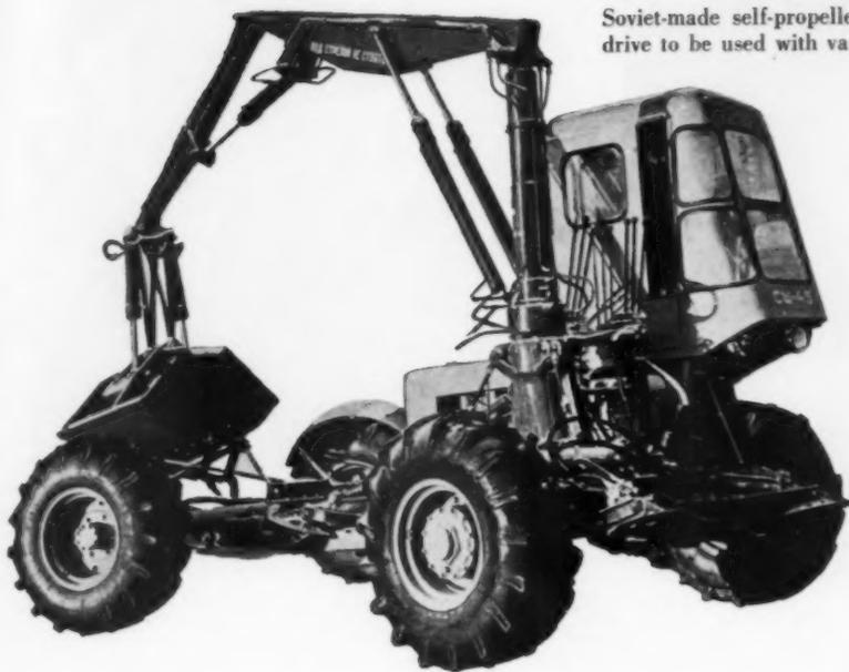
Soviet-made self-propelled chassis with four-wheel drive to be used with various mounted implements.
