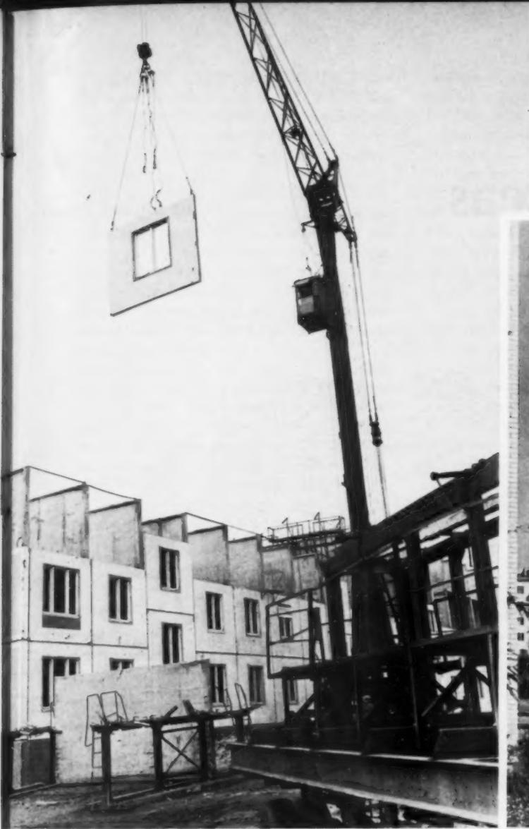
Prefabricated panels are used on a large scale to expedite construction and to reduce building costs. Panels are made at the factory and assembled on the site.
