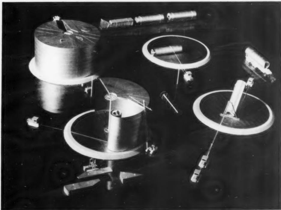
This prefabricated method of constructing oil tanks won a Lenin Prize for Paton Institute engineers. Steel sheets are welded at the plant, carried to the site in rolls and there assembled by machines.
