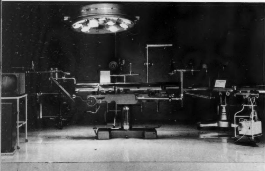
With this multipurpose orthopedic table of new design, a product of Soviet medical engineering, all kinds of surgical operations can be performed, including the placing of a plaster cast, if that is required, without moving the patient. The unit has facilities for X-ray photography and a built-in device that makes it possible to follow the operation on a television screen. The findings of electronic and nuclear physics research are built into most of the currently designed medical units.
