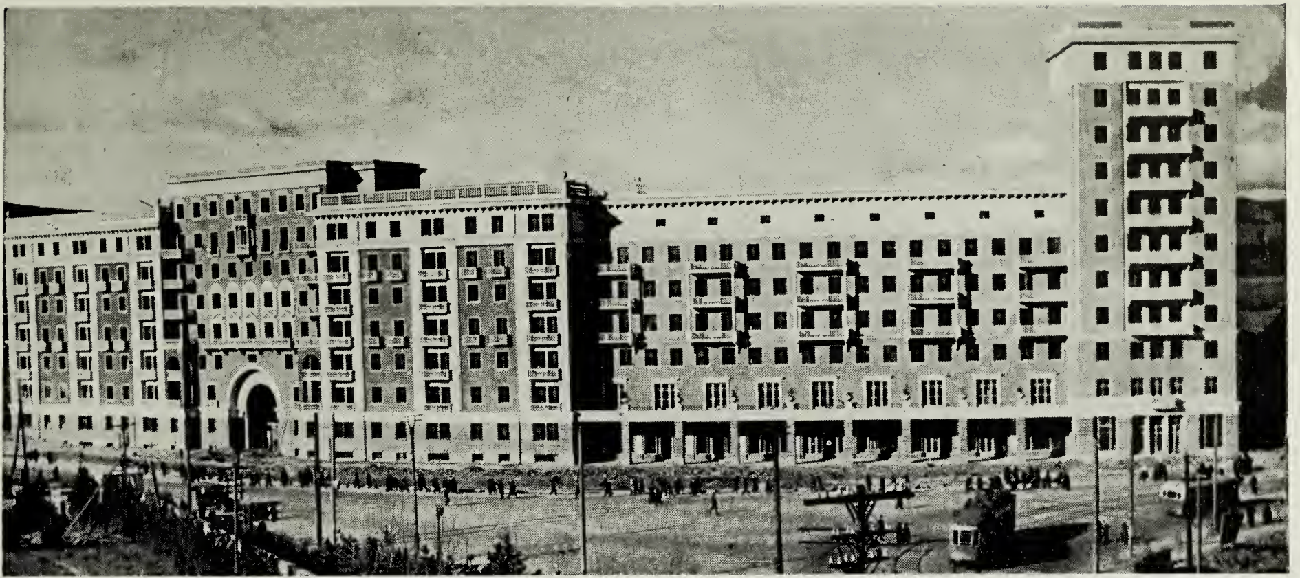
TBILISI—the Square of Heroes and a new apartment house.
