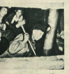
The use of pneumatic drills in coal-mining must be closely co-ordinated with the work of propping, shovelling and transport.
