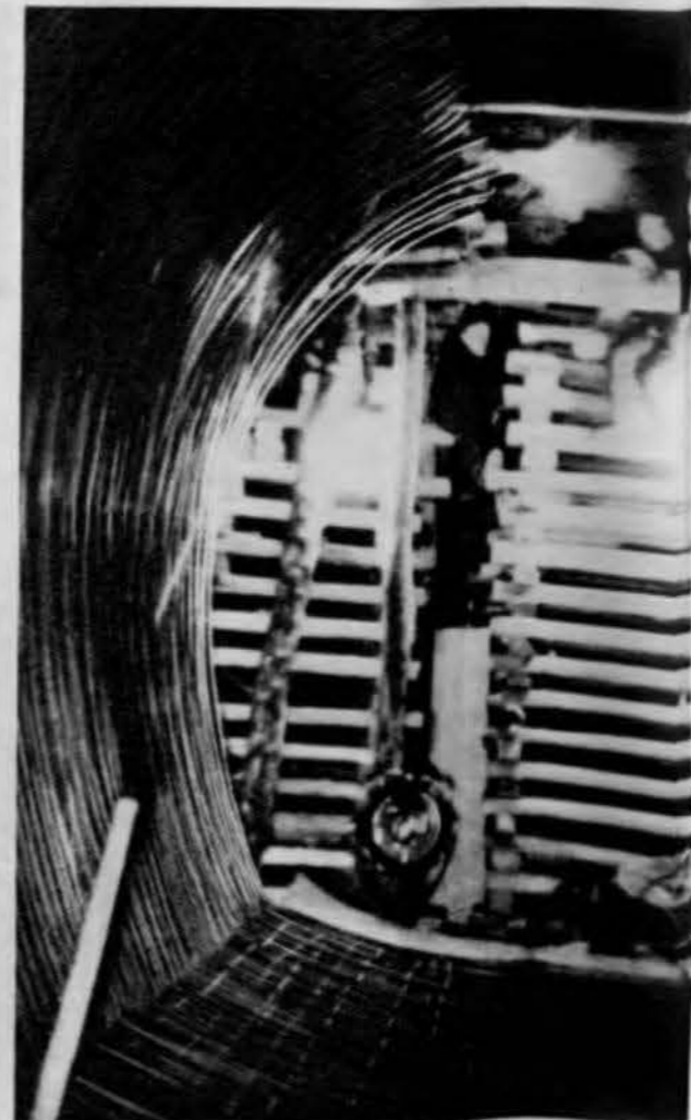
The water-tunnel of the Paisha Reservoir in construction
