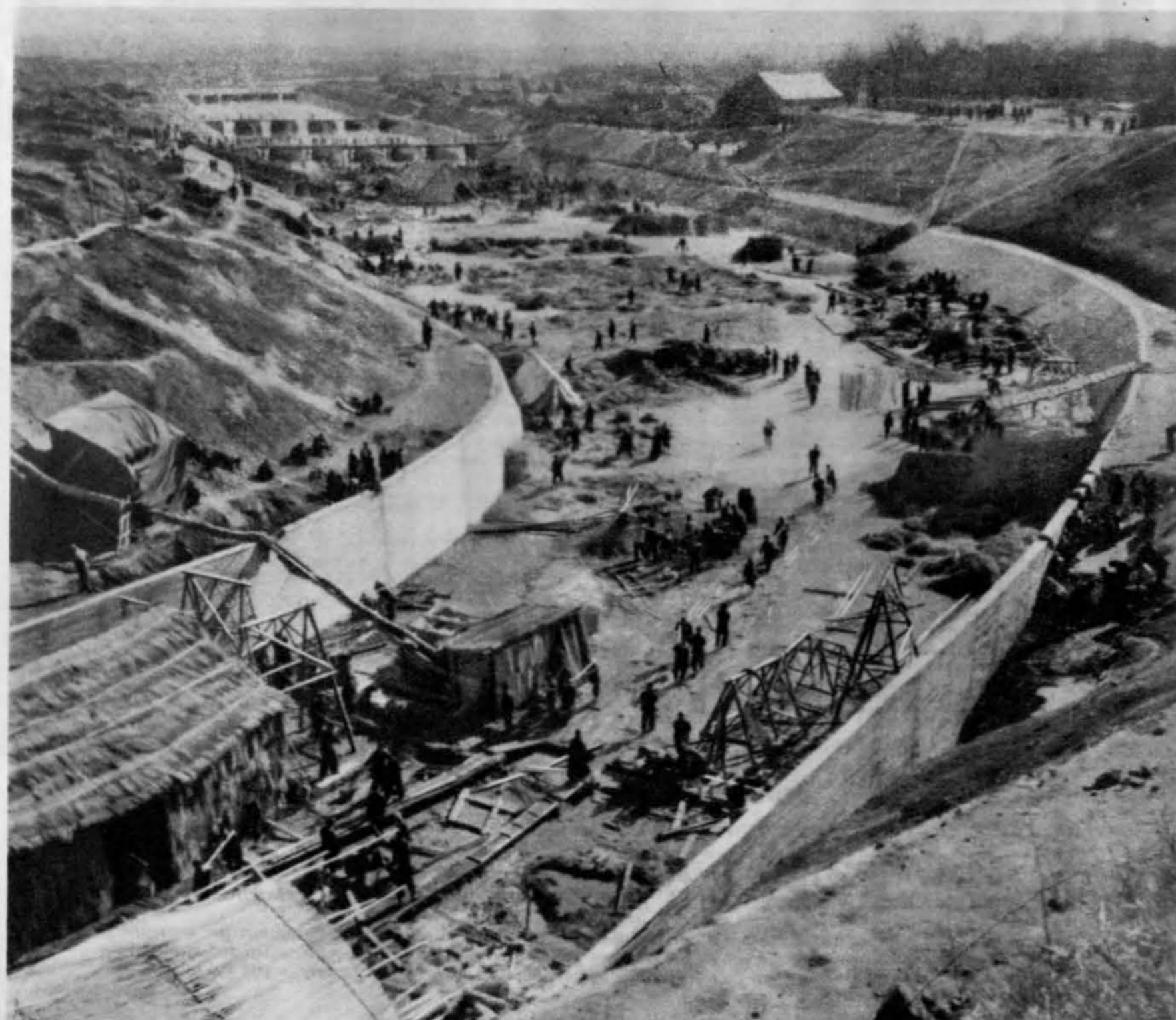
A view of the Paisha Reservoir on the Ying River. The reservoir will be completed before the flood season in 1952
