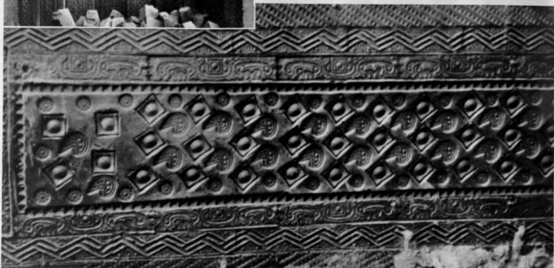
This typical tomb of the Han dynasty is built with hollow bricks of decorative design
