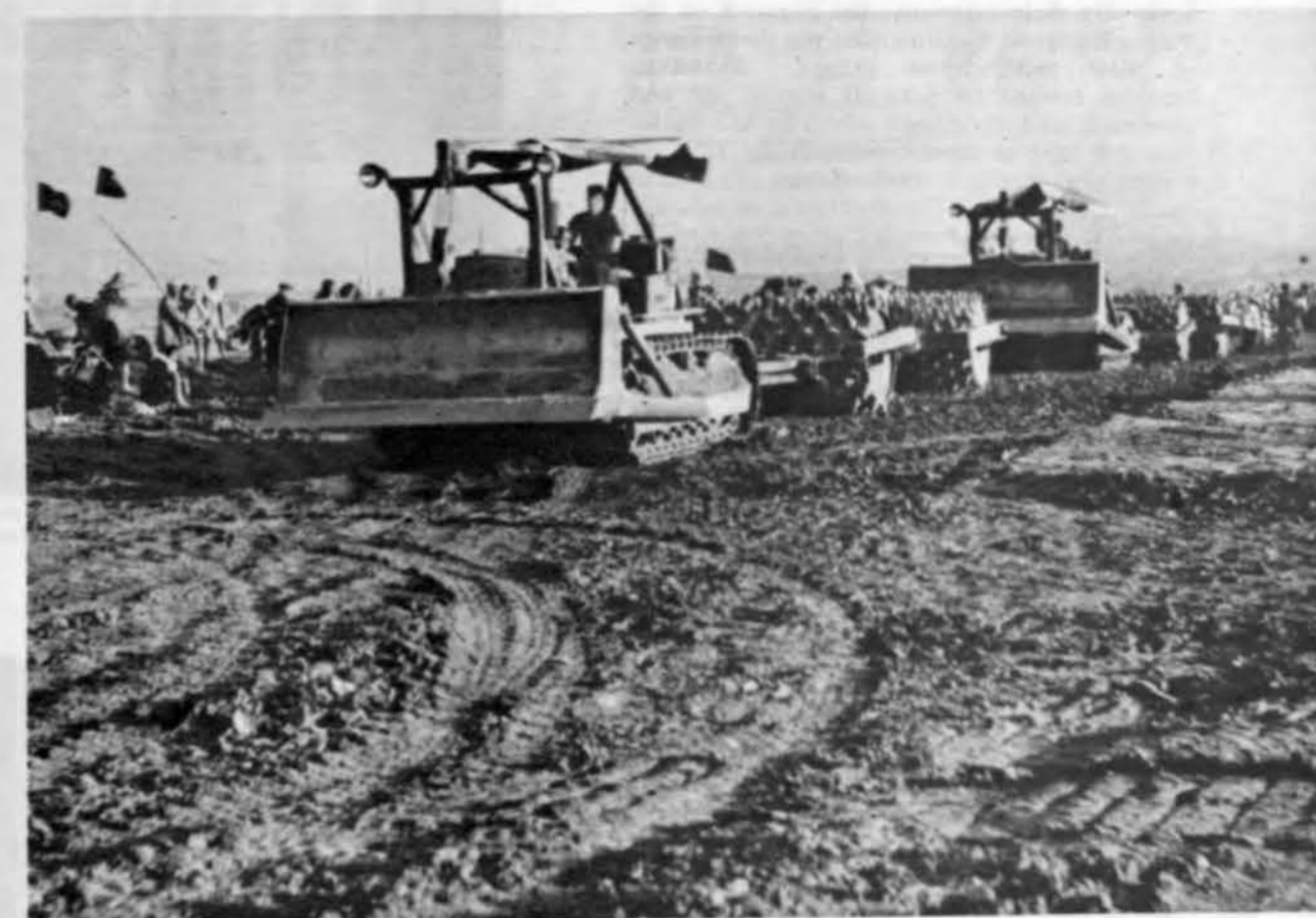
Bulldozers and sheep-foot rollers in action on the dams
