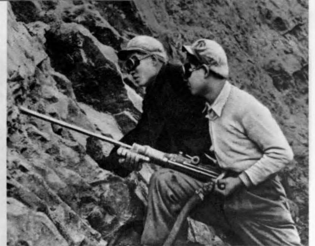
Air-compressors are used for drilling the Paisha tunnel
