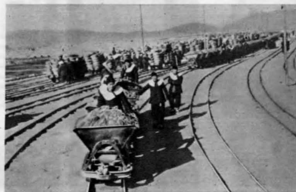
Thousands of trucks on a network of light railways operate an all-day service transporting earth, stones and other material to the dams
