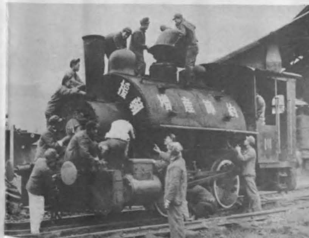
Workers' enthusiasm overcomes transport difficulties—a group of workers in the locomotive repair shop of a Chungking factory constructed this locomotive in their spare time from wreckage and scrap iron left behind by the Kuomintang
