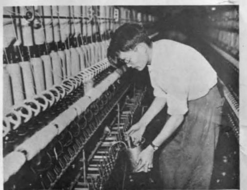
Shanghai textile engineers create national record in cleaning time during the patriotic production movement-Chen Sheng-ming and his team of engineers in a Shanghai textile factory, reduced the time for cleaning a ring frame to only twenty minutes. The new method,
