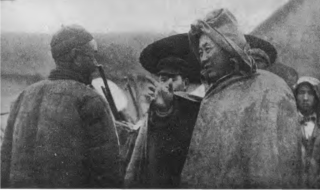
Fu Tso-yi conversing with the local peasants while inspecting the work of the Huai river project.
