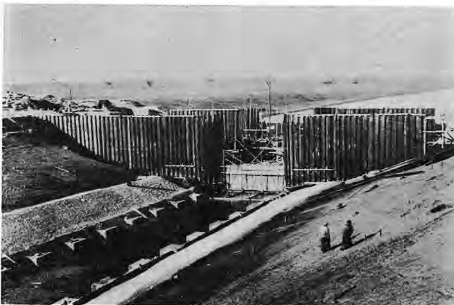
The Huaiyin lock, on the lower reaches of the Huai, is one of 56 locks already completed in the first phase of the Huai river project in 1951.
