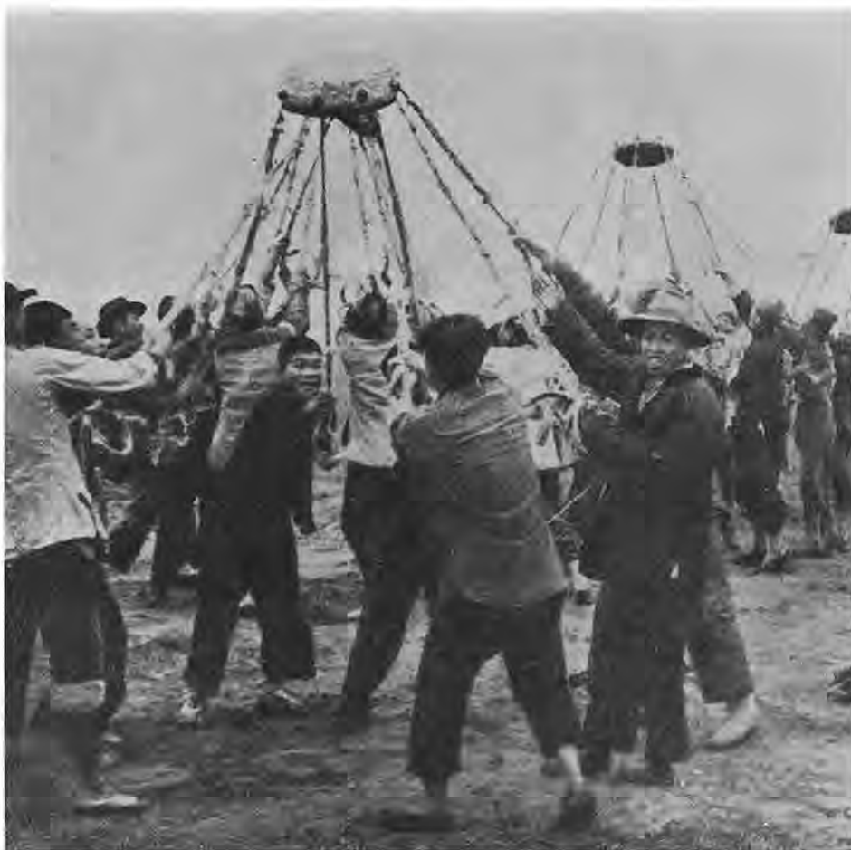
Workers swinging 220-lb. stones to compact earthwork in the traditional Chinese way. Later there will be machines to do this.
