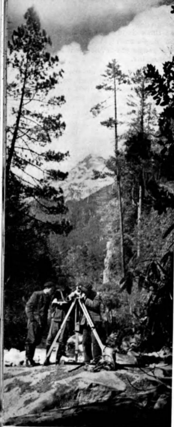
A survey team maps a new hydraulic project in the great forest of Pomi, near the new timber-industry town of Dzamu, built since the liberation.
