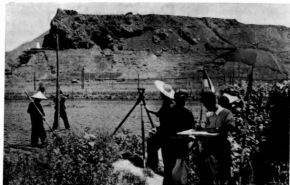
Surveying the iron deposits in Taku Mountain with a view to extending the existing mining area.
