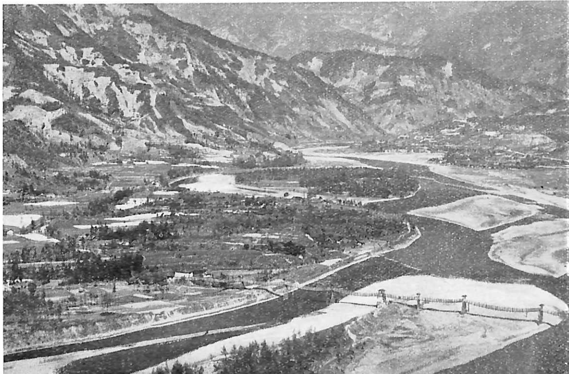
The Tukiangyen irrigation system.
