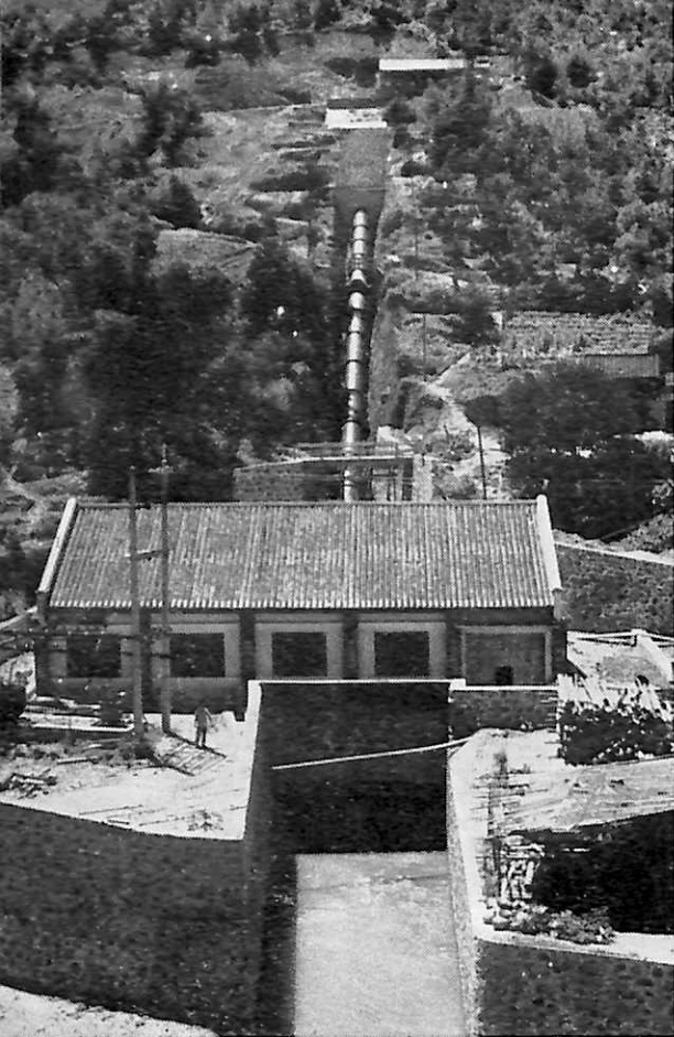
A 1,000-kw. hydroelectric power station at Kuangning county's Tang village.
