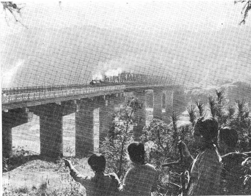
Part of the new Chihcheng-Liuchow line has opened to traffic.
